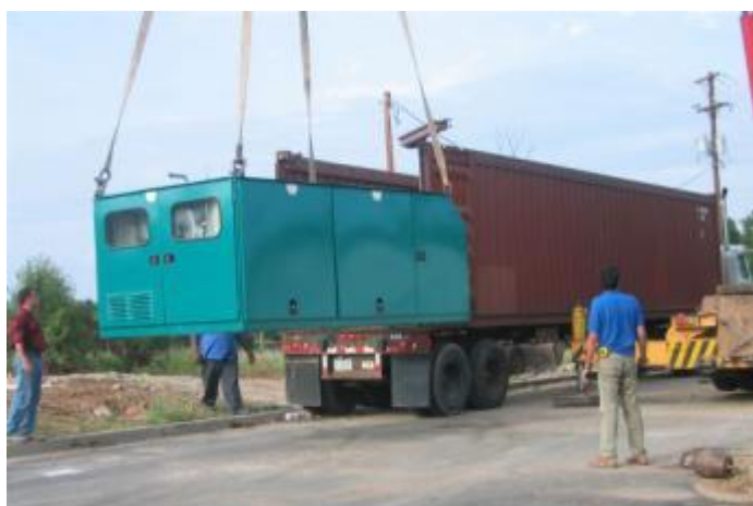
Loading of standard main winch
